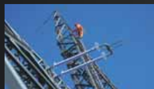
Berlin Electricity, Germany
